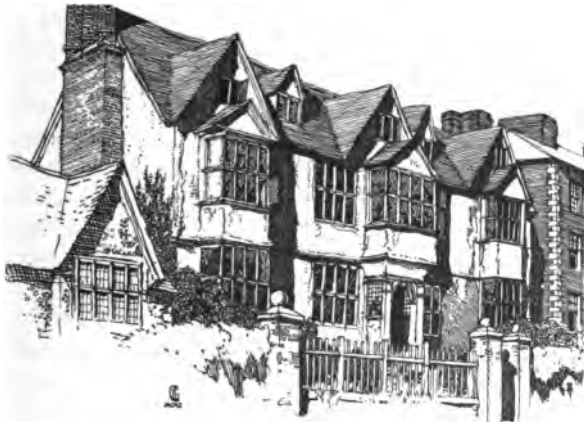
Egerton House, Berkhamstead St. Peter.
